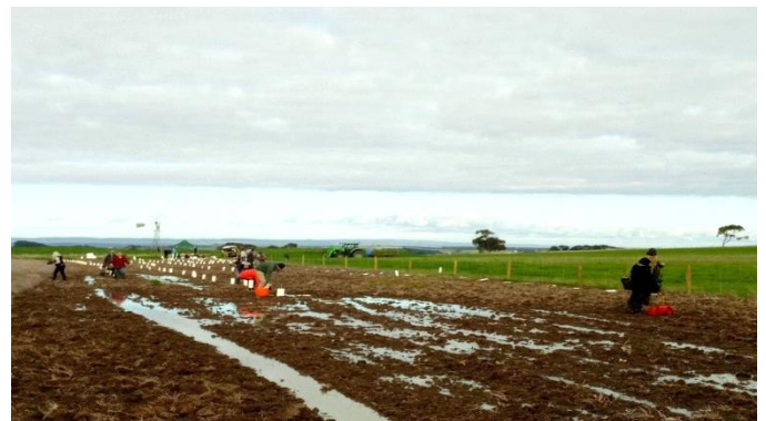
Recreating wetland habitat at Buckley
