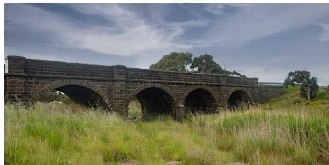
The historic Rothwell Bridge
